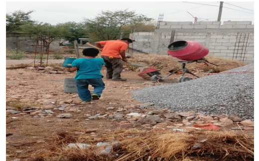
Ten Construction and expansion projects in 12 different states
