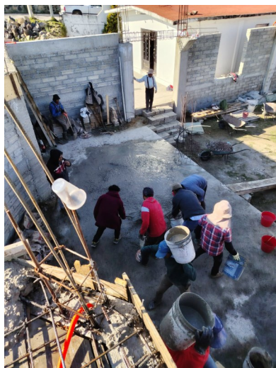
Takes a lot of concrete to build
