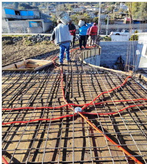
Getting roof ready at San Felipe. We have seven more projects.
