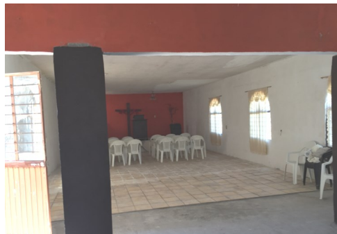
REMODEL AND EXPANSION AT THE CONSTANOS CONGREGATION
